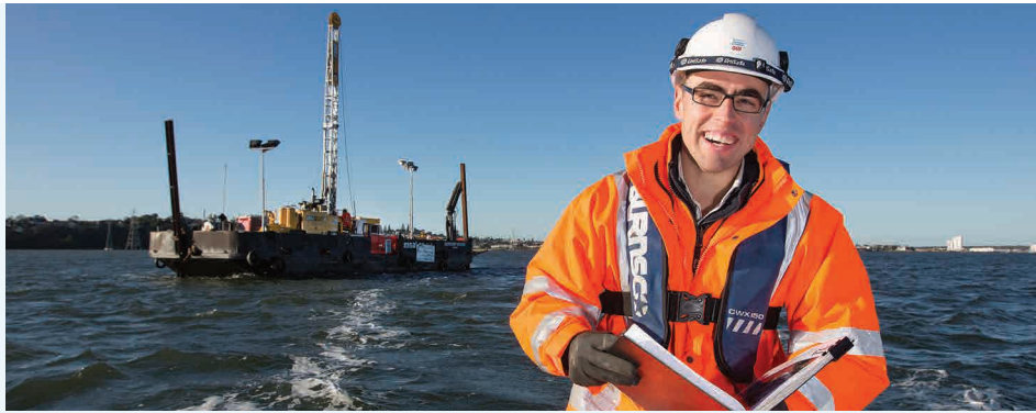
Pictured above: Watercare engineer Bojan Jovanovic monitors geotechnical investigations on the Manukau Harbour. A series of 120mm-wide boreholes is being drilled 45 metres below the seabed along the proposed tunnel route.
